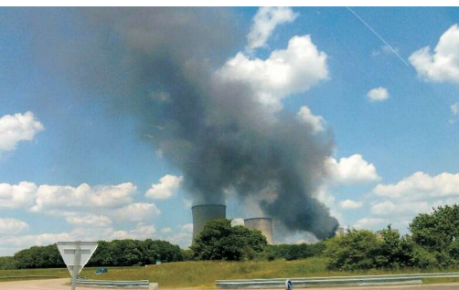
7.6.2013: Brand Transformator Block 1
